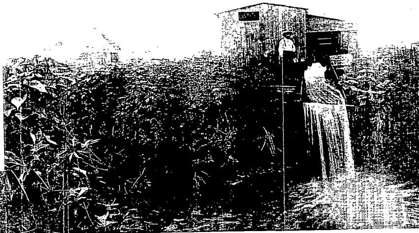
An artesian well north of Columbus, on the Grathern farm, Platte County, Nebraska. Before adequate pumping technology was developed, groundwater had to be raised by buckets or flow to the surface as a result of the pressure of a confining layer of sediment or other sufficient pressure head. Photo courtesy of Nebraska State Historical Society.
