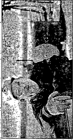
LEFT: Jim Foster of Burdon Well Drilling in Bartley, Neb., welds part of an irrigation well on a farm near Trenton.
