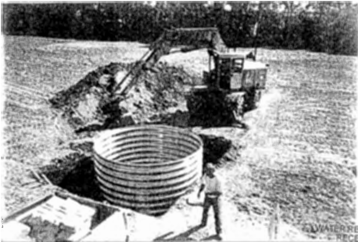
Photograph I-4: Infiltration Test Pit Construction
