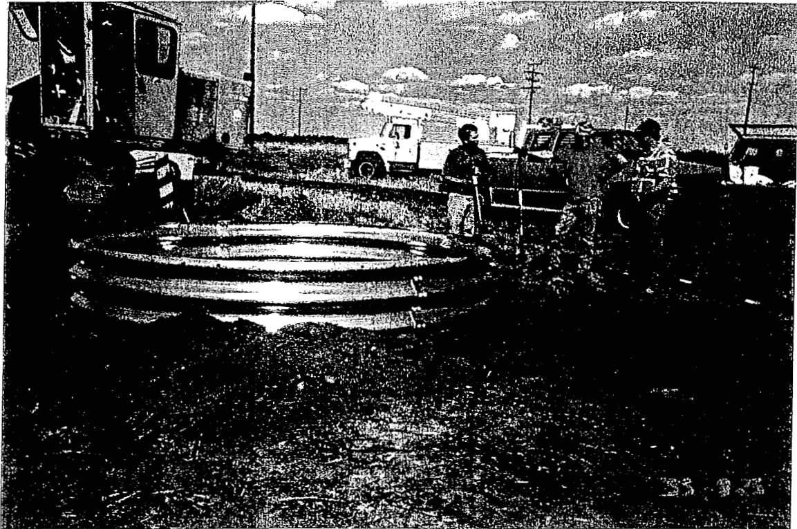
Photograph I-5: Infiltration Test Pit Construction
