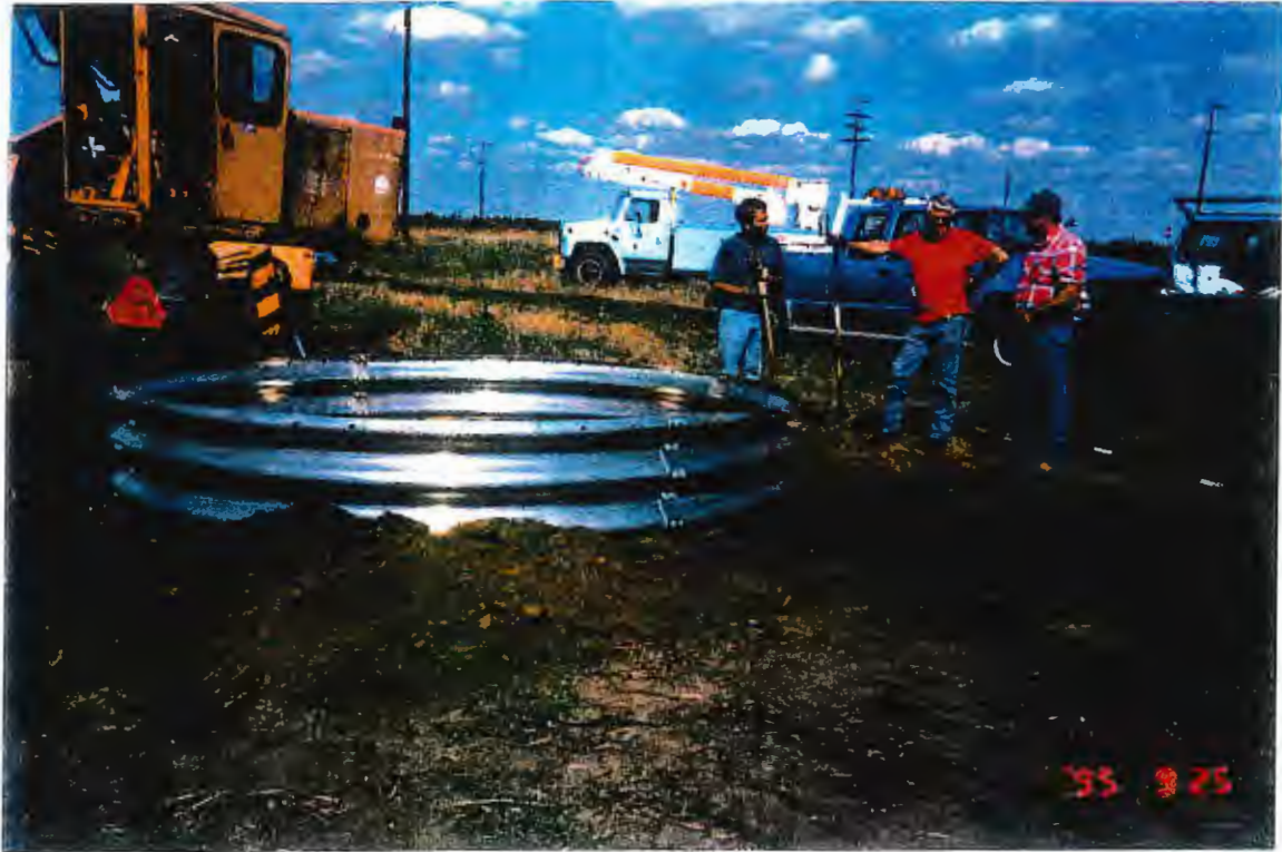
Photograph I-5: Infiltration Test Pit Construction
