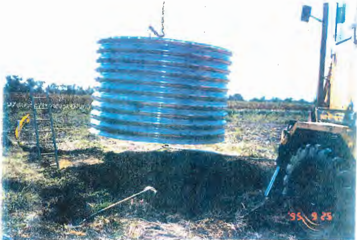
Photograph I-3: Infiltration Test Pit Construction
