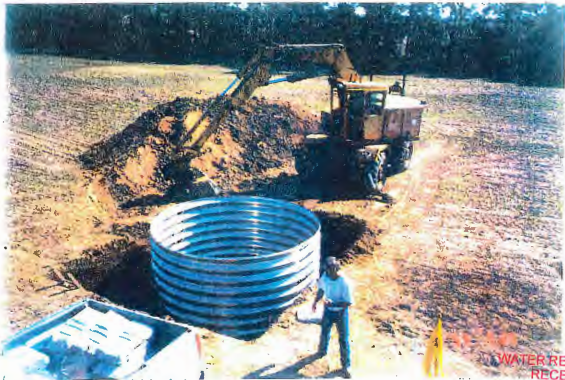
Photograph I-4: Infiltration Test Pit Construction
