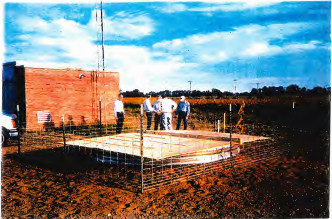
Photograph I-6: Infiltration Test Pit Construction
