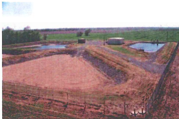
Example of Recharge basin
