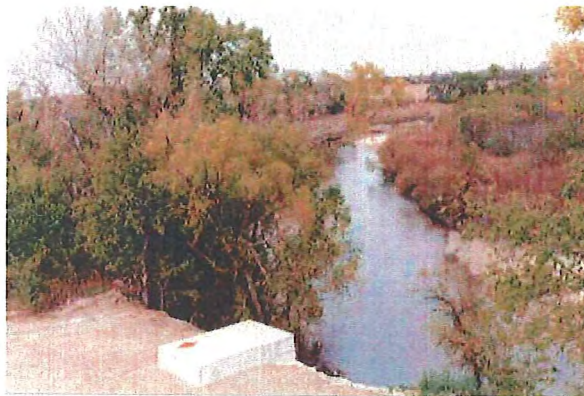
Example of Intake Structure on the Little Arkansas River
