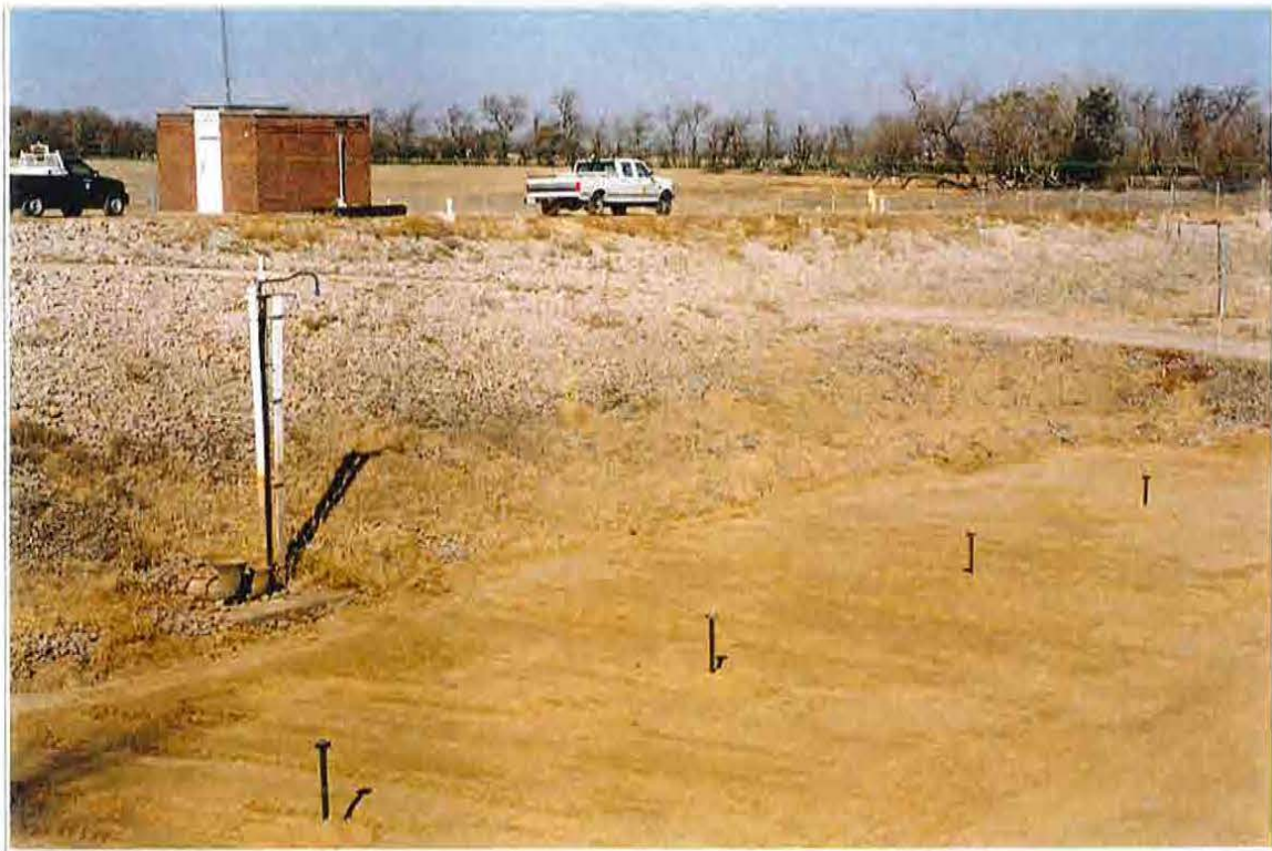
Recharge Basin with Gravity Recharge Wells - Halstead Recharge Site November 17, 1999
