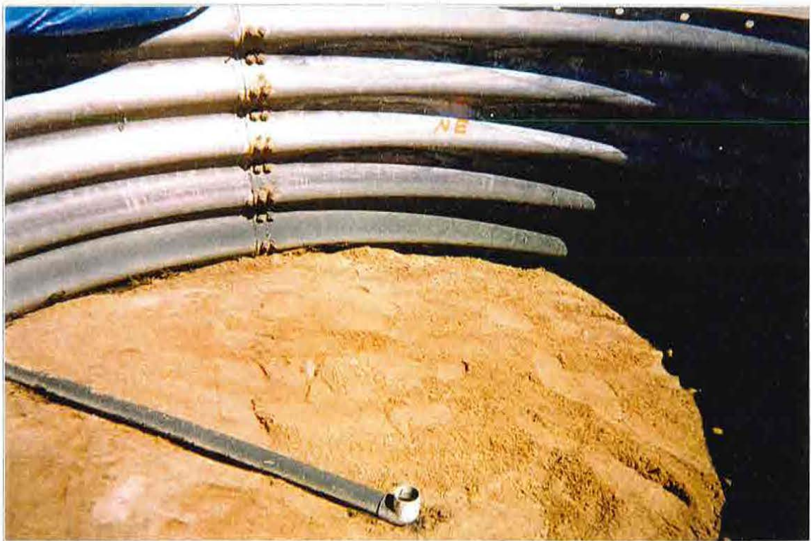
Floor of Simulated Surface Water Recharge Trench Sedgwick Recharge Site
