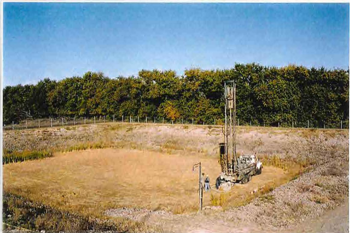
Installation of Gravity Recharge Wells - Halstead Recharge Site October 20, 1999
