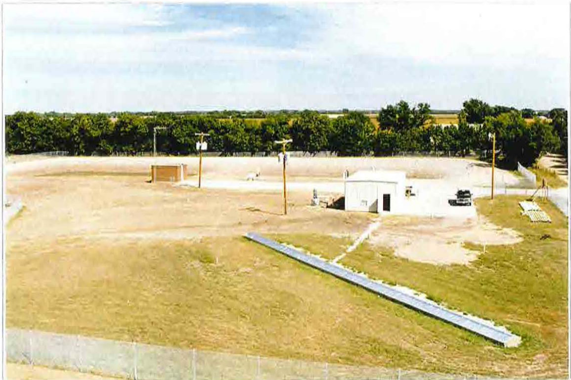
Recharge Trench and Well - Halstead Recharge Site September 17, 1997
