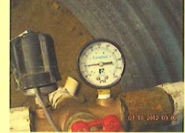
Newly installed pressure gauge during Test#1
