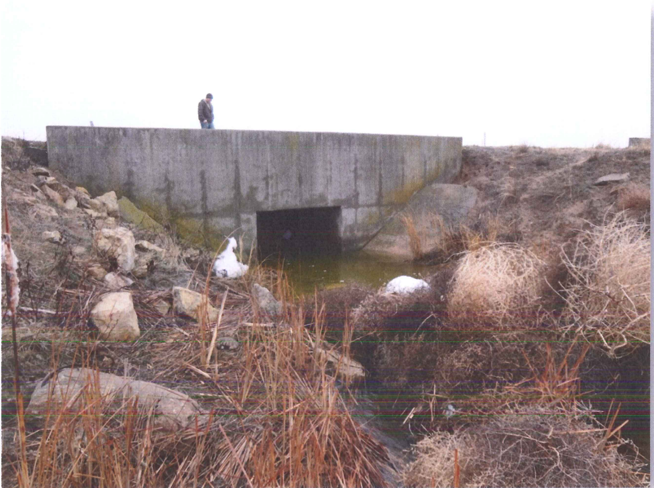
9: Water Control Structure DCA.
