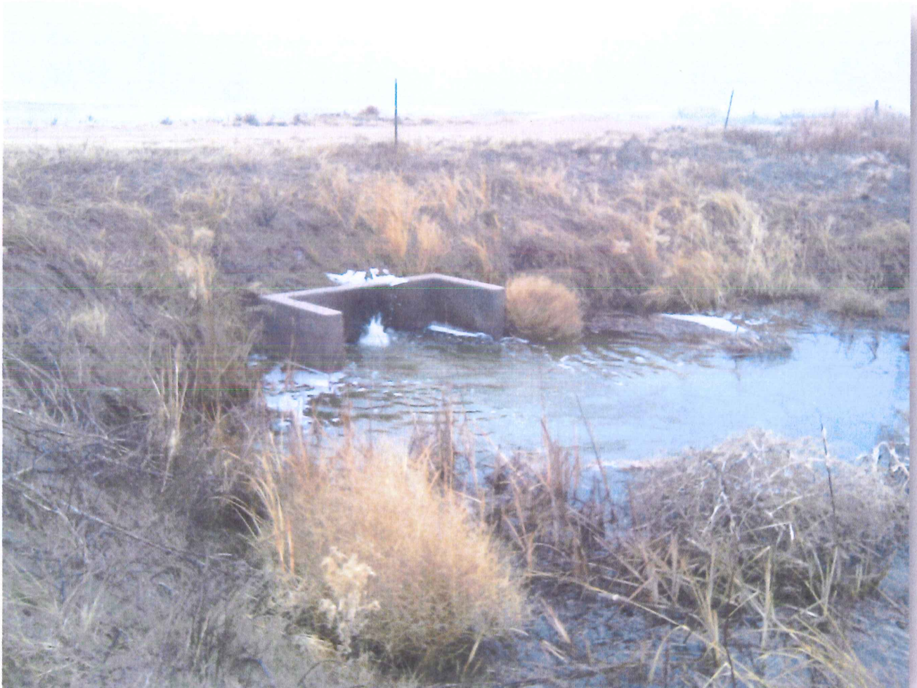
8: Downstream Culvert at Water Control Structure 24C.
