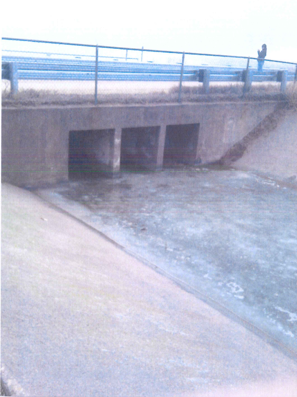
4: Downstream Apron at Water Control Structure A1.
