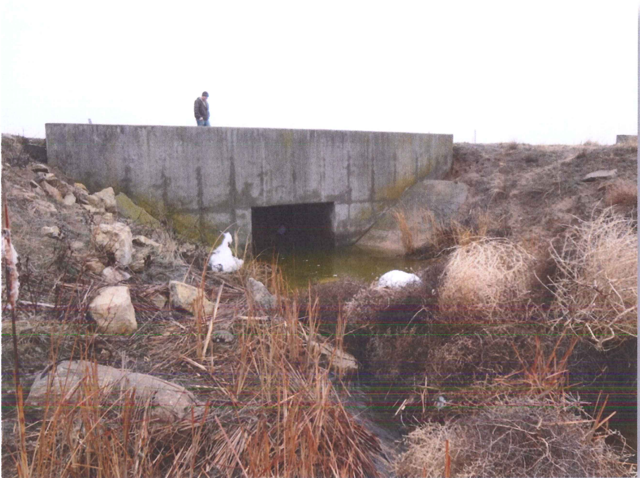
9: Water Control Structure DCA.
