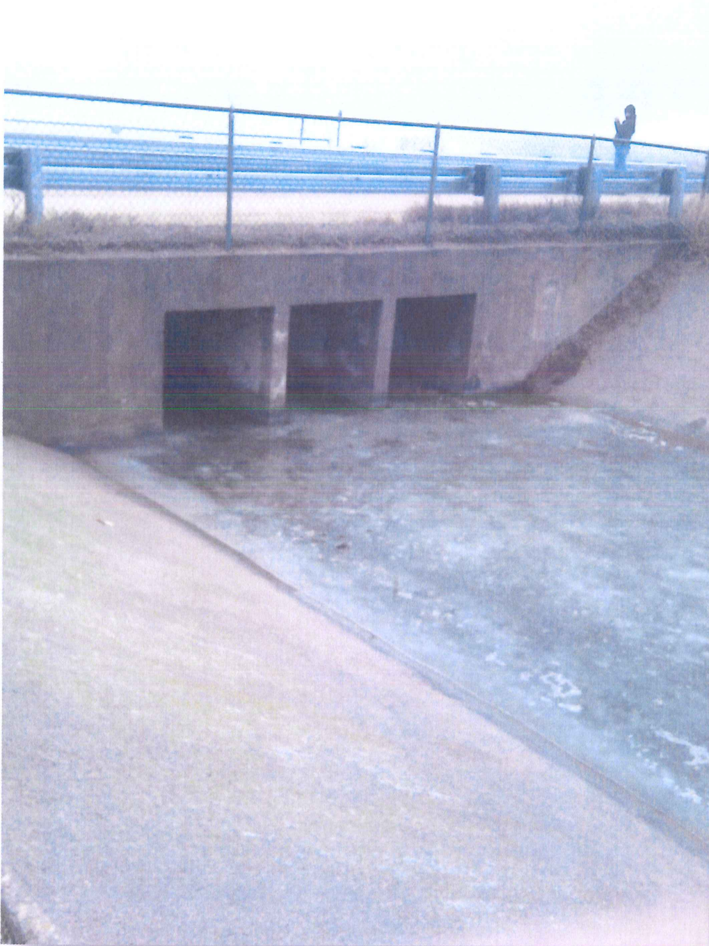
4: Downstream Apron at Water Control Structure A1.
